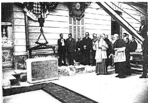
Laying the foundation stone - 20 April 1929
