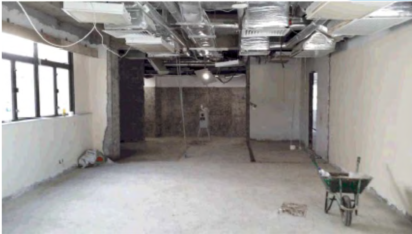
Building Works in Progress
