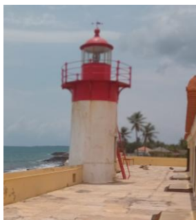
Figure 38 - Lighthouse of Ilhéu Rei
