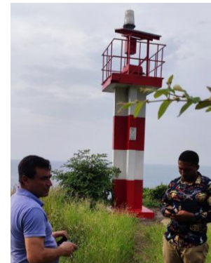
Figure 9 – Visit to a light house in Lagoa Azul
