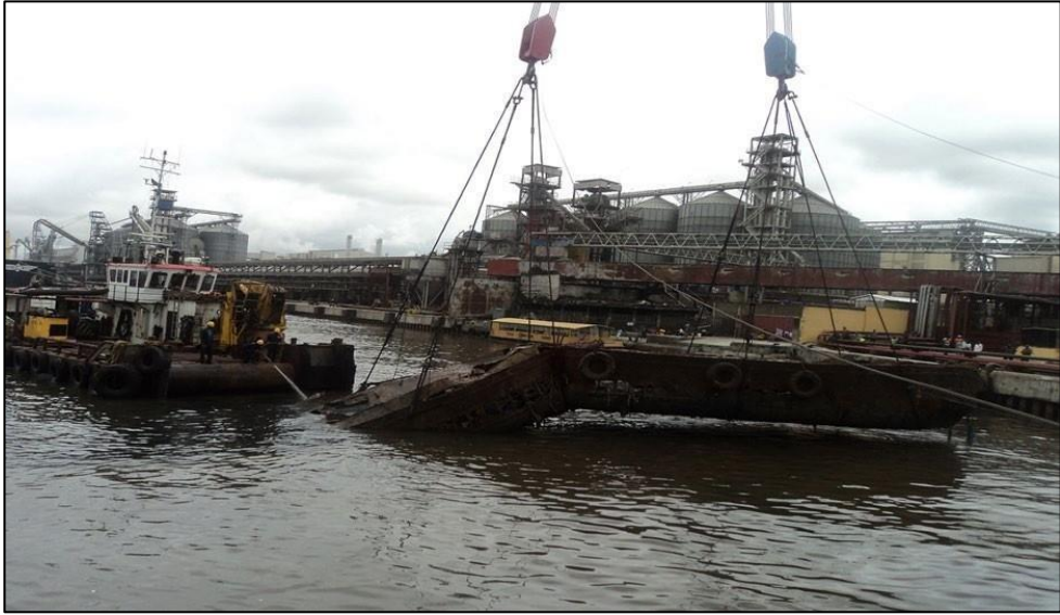
Figure 1. Dredging and wreck removal in Lagos Channel.
