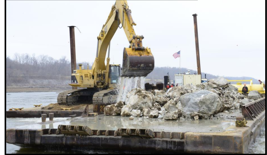
Rock Pinnacle removal at Thebes, IL
