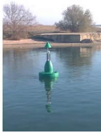
MANGALIA HARBOR BEACONING SYSTEM
