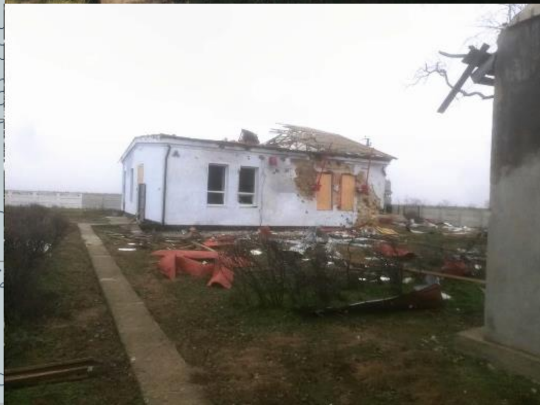
Serves for the household needs of the lighthouse staff, as well as for the backup diesel generators exploitation.
