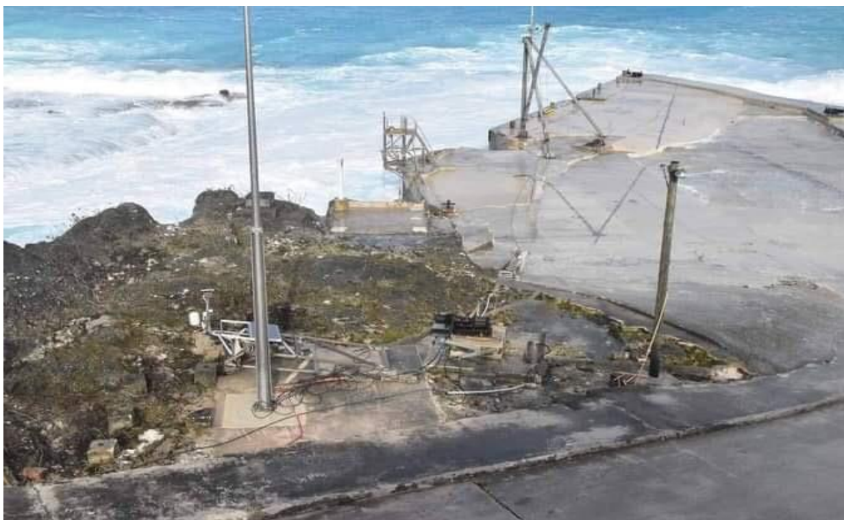
Figure 4. Photo of the tide gauge hut and mast, GNSS sensor and tide gauge mount after TC Tino 17 th January 2020.
