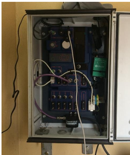
Figure 5: Cabinet of digital tide gauge installed in Nacala Port
