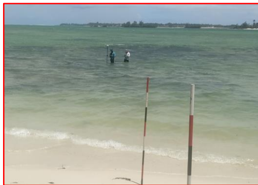
Figure 6: Pole Sounding at Surinam
