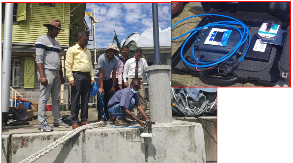
Figure 11: Commissioning of ATG
