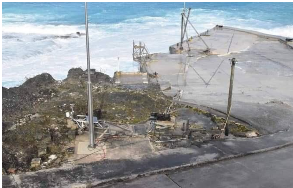
Figure 4. Photo of the tide gauge hut and mast, GNSS sensor and tide gauge mount after TC Tino 17 th January 2020.
