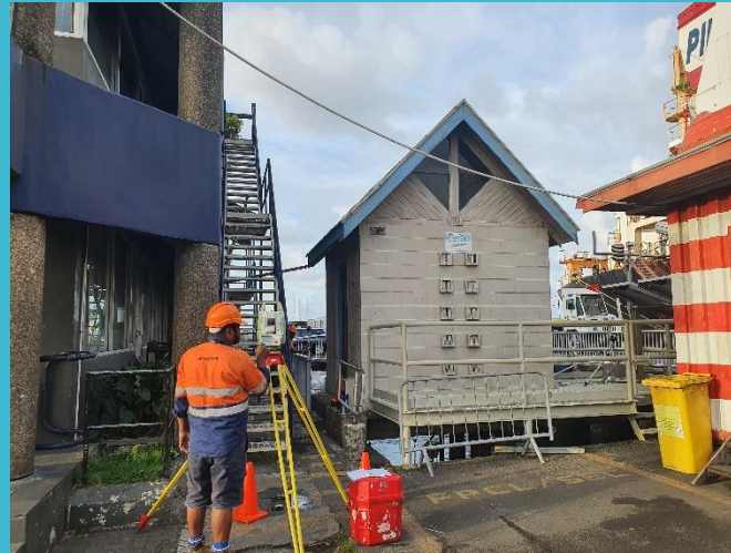
Suva Tide Gauge Station Connection to GNSS CORS
