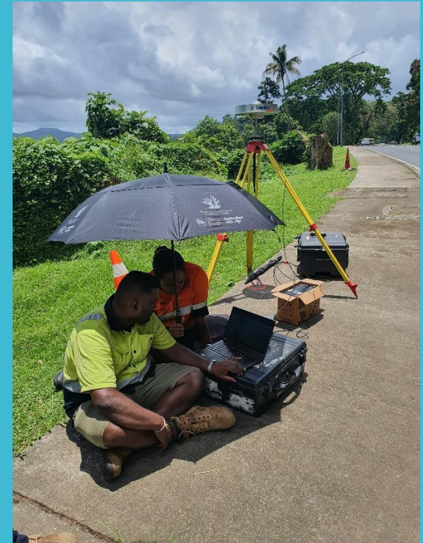
Geodetic Control Survey Static GNSS for Suva Network
