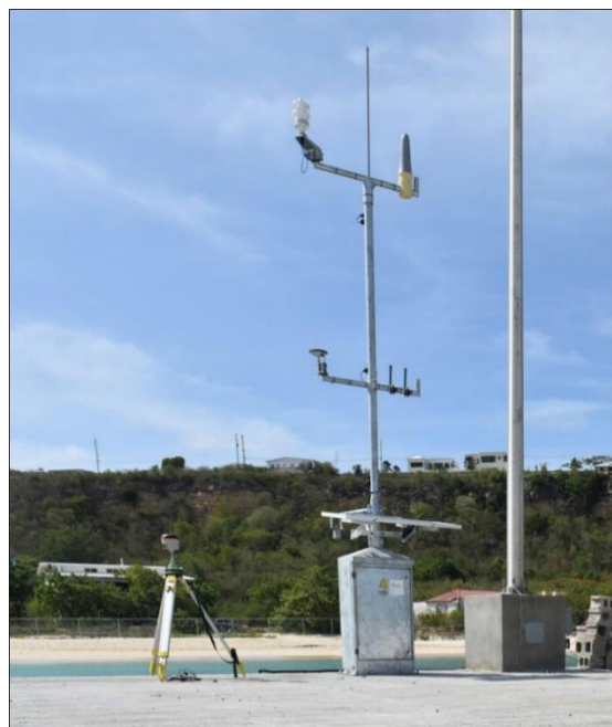
MEMS installed on Road Bay jetty Anguilla.
