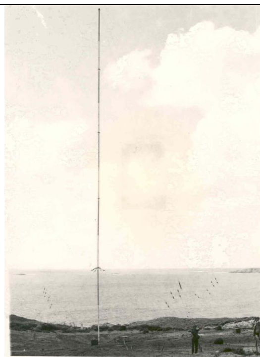
Late 1940s to mid 1990s: Shore based electronic position fixing systems could achieve accuracy typically between 20 – 100 metres compared to GNSS on modern ships.
