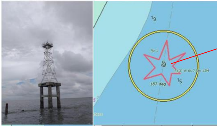
Lattice beacon with Height less than 10 meters.
