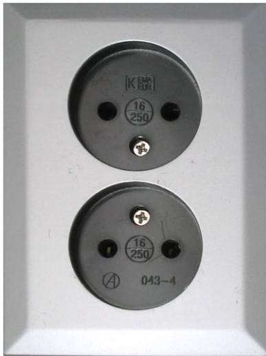
The standard 2-wire plug used in Class II, unearthed, applications is popularly known as the Europlug, which is described in CEE 7/16. It will mate with any socket that accepts 4.0–4.8mm round contacts on 19mm centres.
